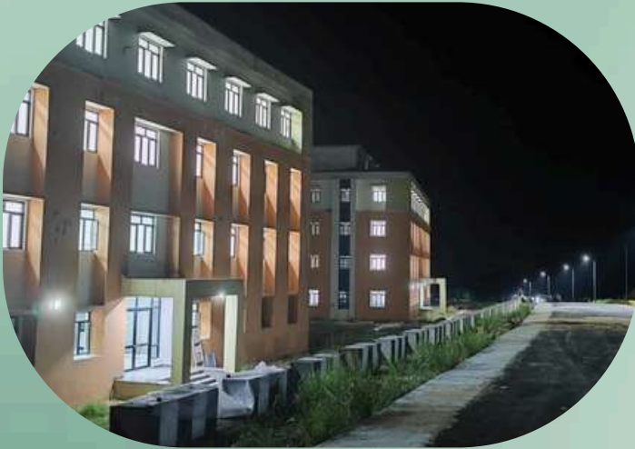
Block C and Block D
